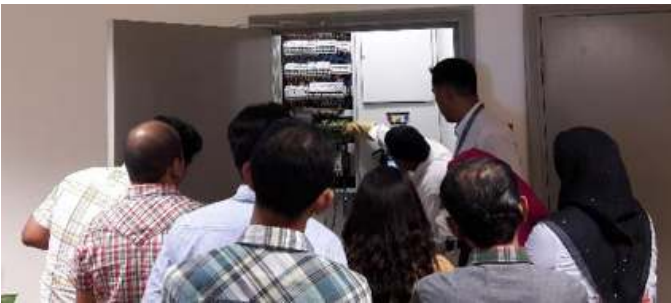
Hands-on activity on energy auditing during technical training on Energy Management and Energy Audit in Building for commercial sector (5 th - 6 th March 2018)
