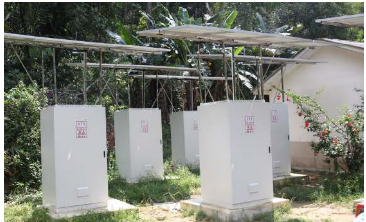
Part of the solar system which has been completed
