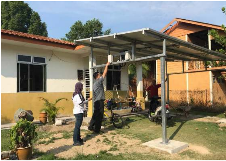
On-site Verification on solar installation at Perak on 14 th May 2018
