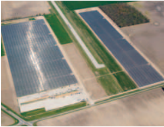
12 MW Wyandot Solar Farm; credit: PSE&G
