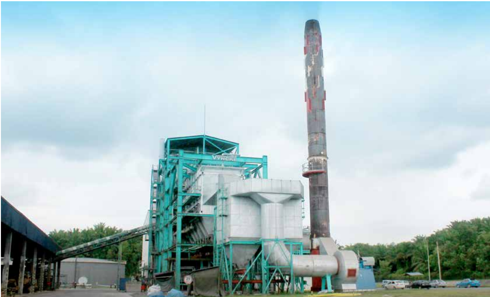
Janakuasa Biojisim 11.5 MW, Kina Biopower Sdn Bhd, Sandakan Sabah. / 11.5 MW Biomass Power Plant, Kina Biopower Sdn Bhd, Sandakan, Sabah.
