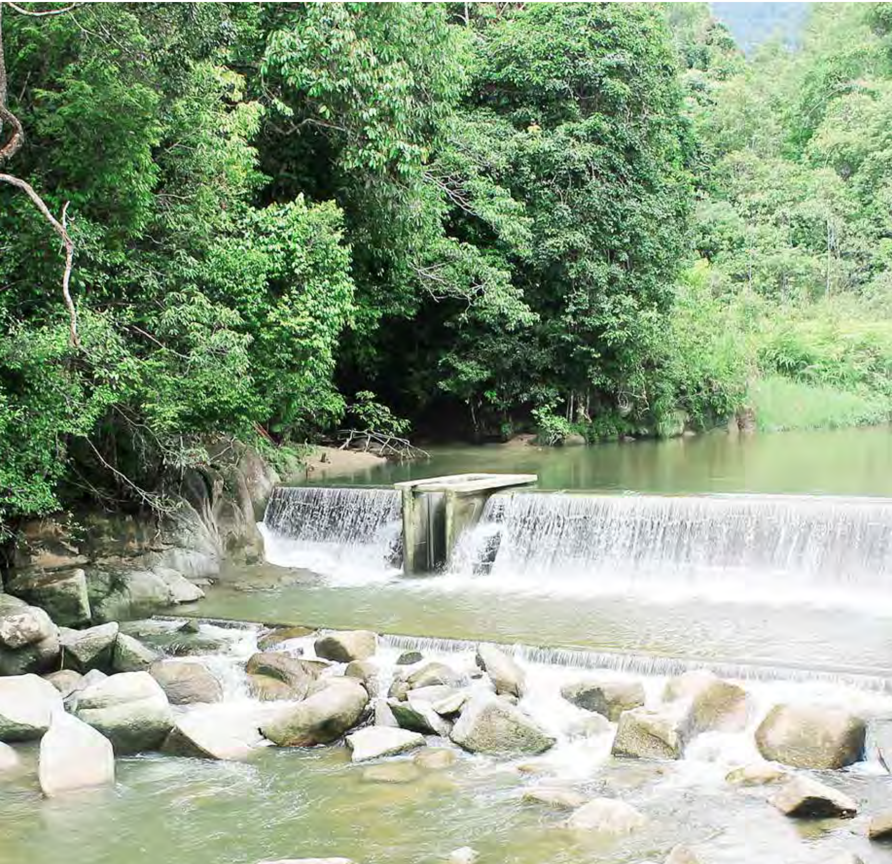
Hidro Kecil 6 MW, Amcorp Perting, Bentong, Pahang / 6 MW Small Hydro, Amcorp Perting, Bentong, Pahang
